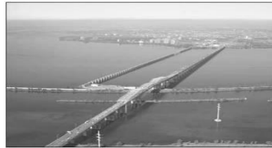
Figure 14 view for existing Champlain Bridge (15)
