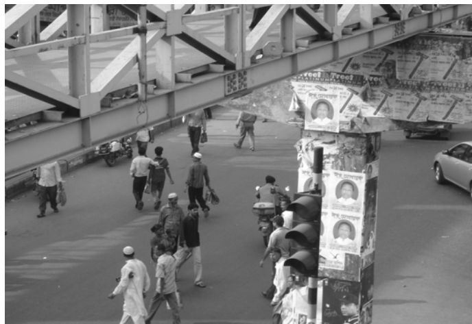
Figure 7: Under Utilization of Overpass
