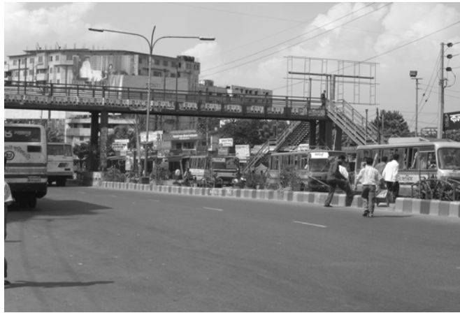
Figure 8: Inadequate Median Barriers
